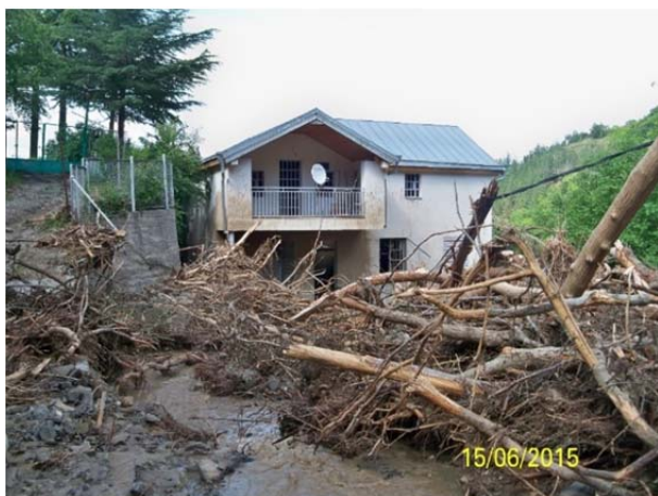
Figure 7 – Debris.mudflow in Tbilisi (Photo G. Gaprindashvili)
