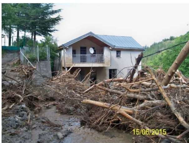
Figure 7 – Debris.mudflow in Tbilisi (Photo G. Gaprindashvili)
