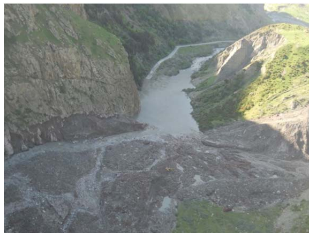
Figure 6 – Blocked Tergi river and created reservoir (Photo M. Gaprindashvili)
